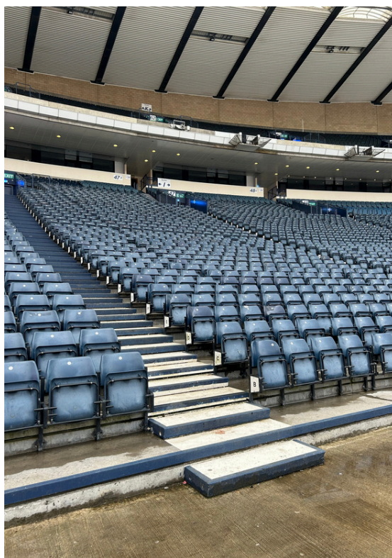
Section I stairs from ground level
