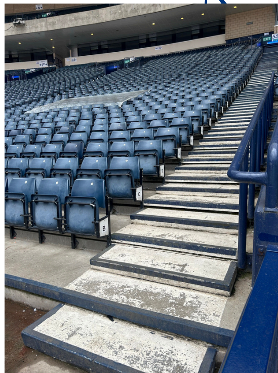
Section P stairs from ground level
